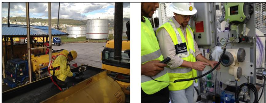
**Figure 4.** Marking of fuels is carried out either manually (left) or by automatic injectors (right).
