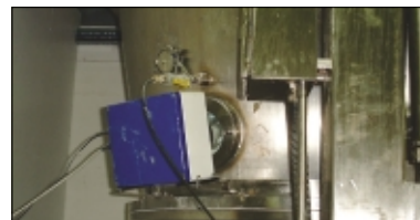
Figure 1. Reflectance near infrared analyser monitoring a fluid bed dryer.
