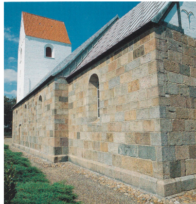
Figure 3. “Asp Kirke”, Jutland, typical medieval Romanesque church illustrating the diverse assembly of hewn rock types. Note later improvement (enlargement) of windows, later lead roofing and addition of a bell tower.
